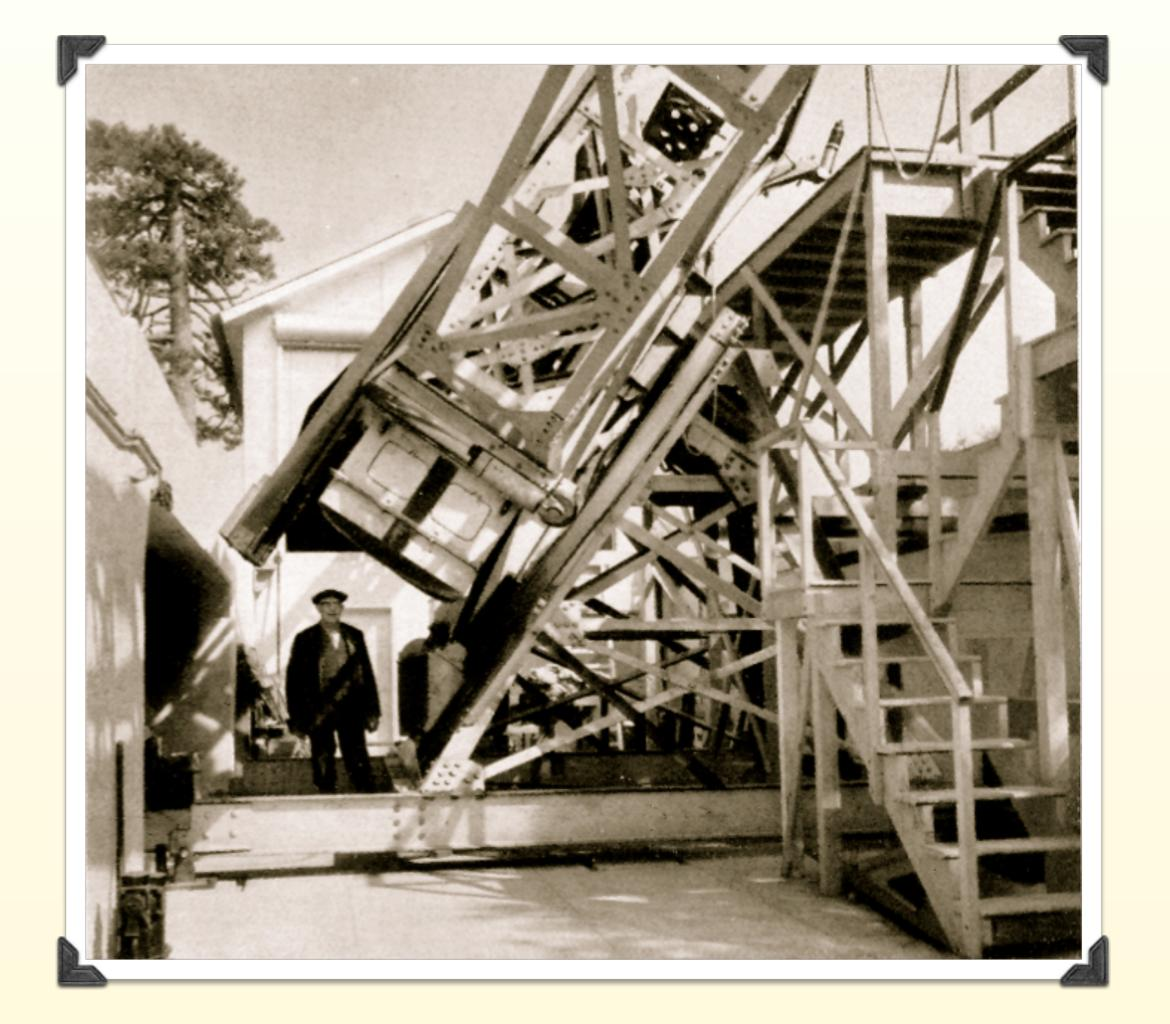
The structure was not stiff enough to maintain the alignment of the interferometer while it was tracking the star (no delay line). Wind excited vibrations that made the visual estimation of the fringe contrast imprecise. Adverse polarization effects probably also played a role.
